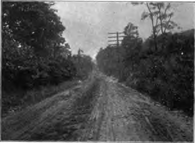
Navesink road, near Stone Church, Monmouth Co., before work was commenced.
